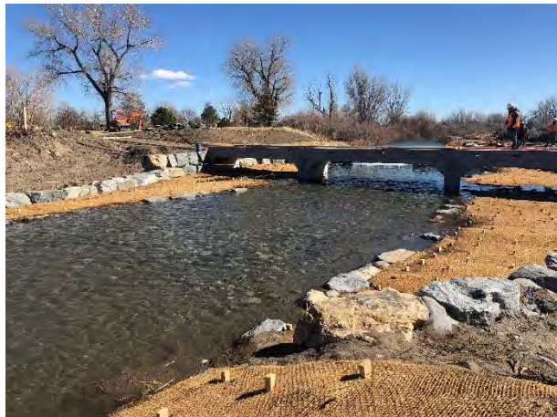
Photo 10 – Constructed Channel @ Golf Cart Bridge
