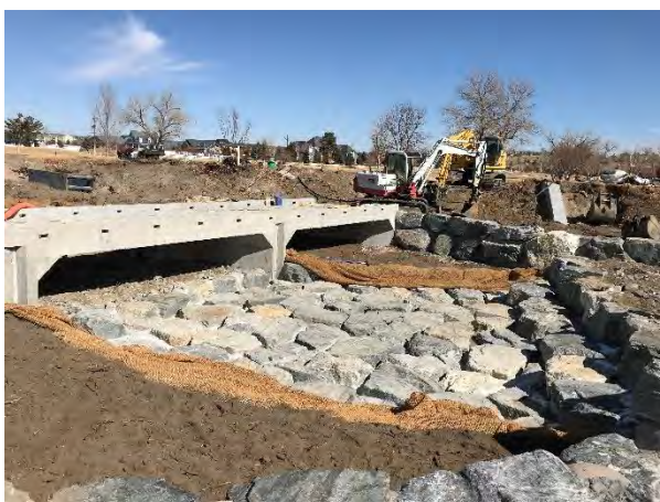
Photo 7 – Grouted Boulder Drop Construction
