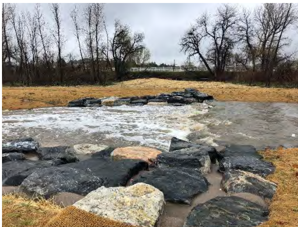
Photo 9 – Constructed Grouted Boulder Drop
