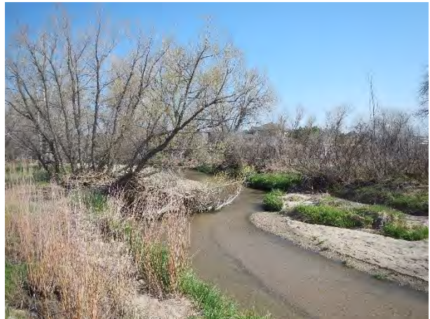
Photo 3 - Typical Pre-project Condition
